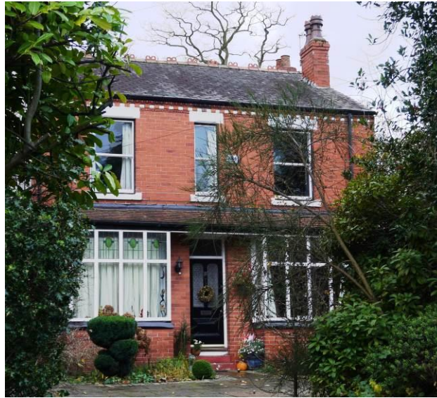
Example of the historic decorative materials such as ridge tiles, terracotta and stained glass
