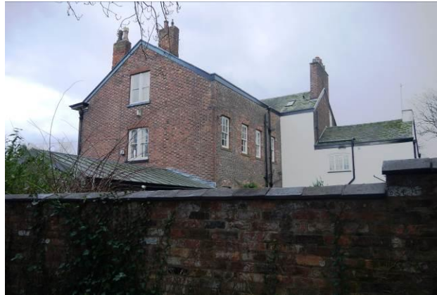
The rear elevation of Ashton New Hall
