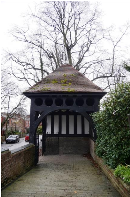
The Lychgate has timber-framing, iron gates and a tiled pyramidal roof
