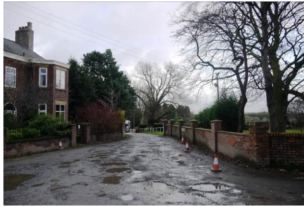
View of the overly large modern brick walls and piers surrounding the paddock and farmhouse
