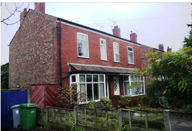
Example of appropriate timber fences and brick walls separating properties. The rear gates are overly large
