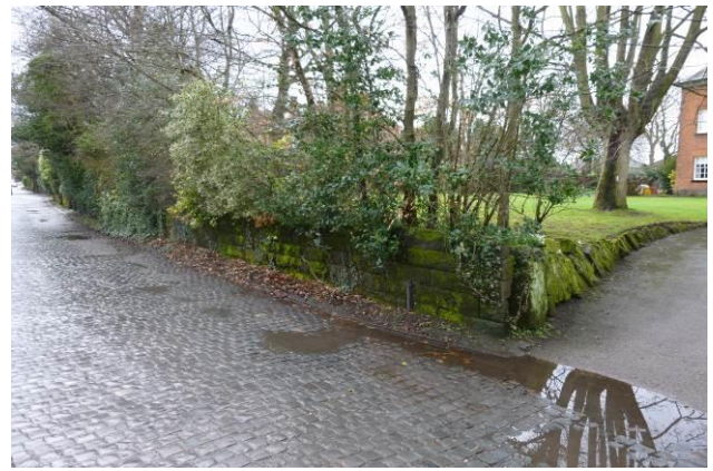
Stone setts on the northern extent of Church Lane within Character Zone A. Note the historic boundary walls and surfaces.
