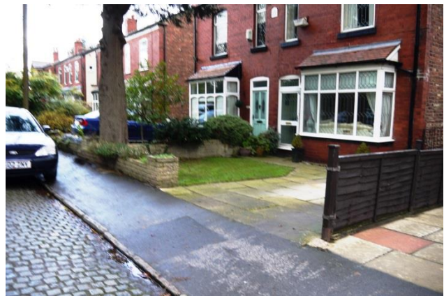
Inappropriate modern materials including concrete slabs and modern stonework. The loss of planting is also detrimental to character
